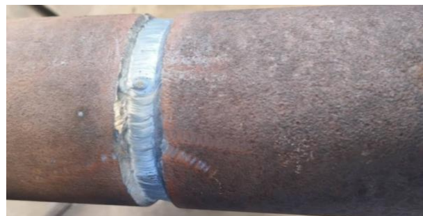
Figure 2: Welded of pipe
