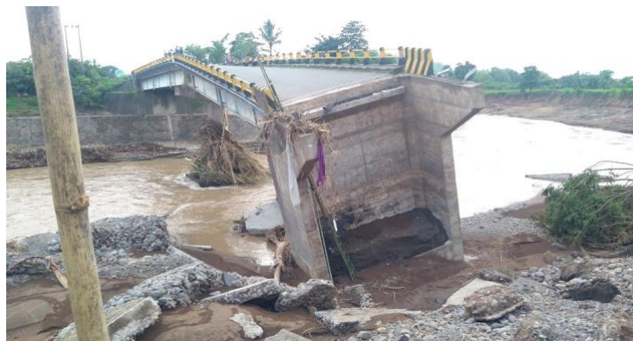
Picture 2. Jenelata Bridge after fall during flood season
