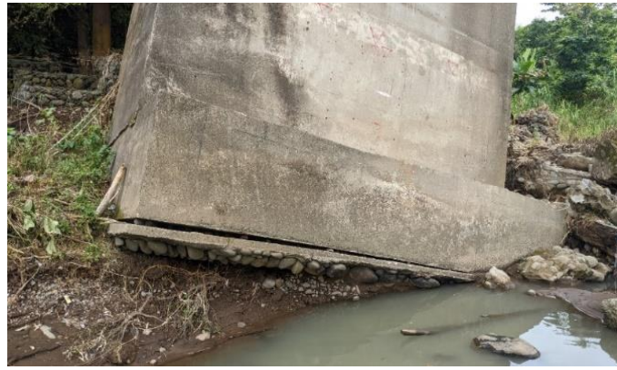
Picture 4. Abutment of Jenelata Bridge
