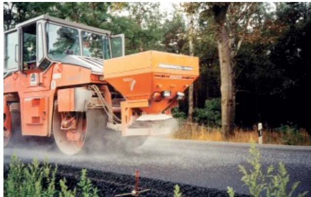
Figure 14. Installation of the gritting material [DAV 2000]
