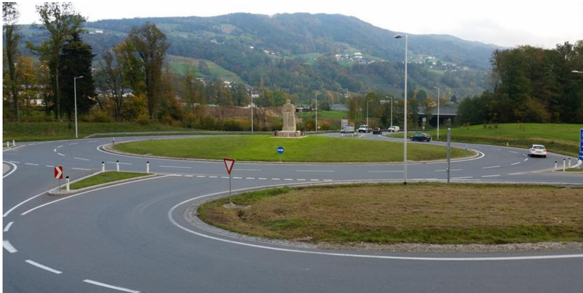
Figure 6. Two-lane roundabout B 154 / highway A1 Mondsee in October 2015 (Hrapović 2020)
