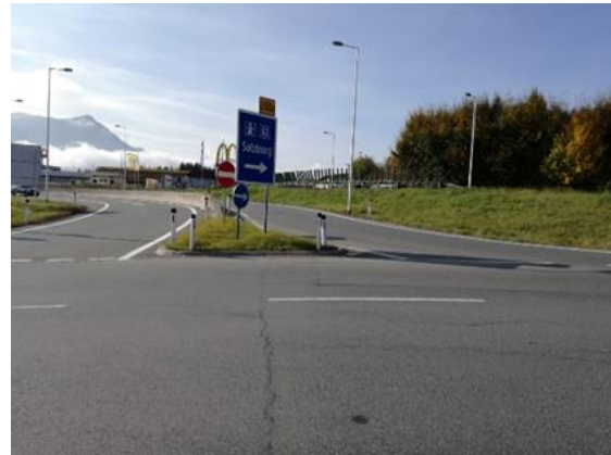
Figure 14. Transverse crack, longitudinal cracks, longitudinal and transverse working seam crack (Hrapović 2020)
