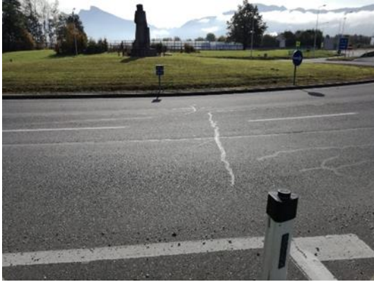
Figure 17. Rehabilitated with hot bitumen compound (Hrapović 2020)
