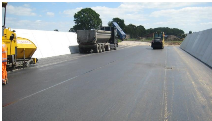
Figure 8. Installation of rolled asphalt in a drive-in silo plant (FGSV 2015)
