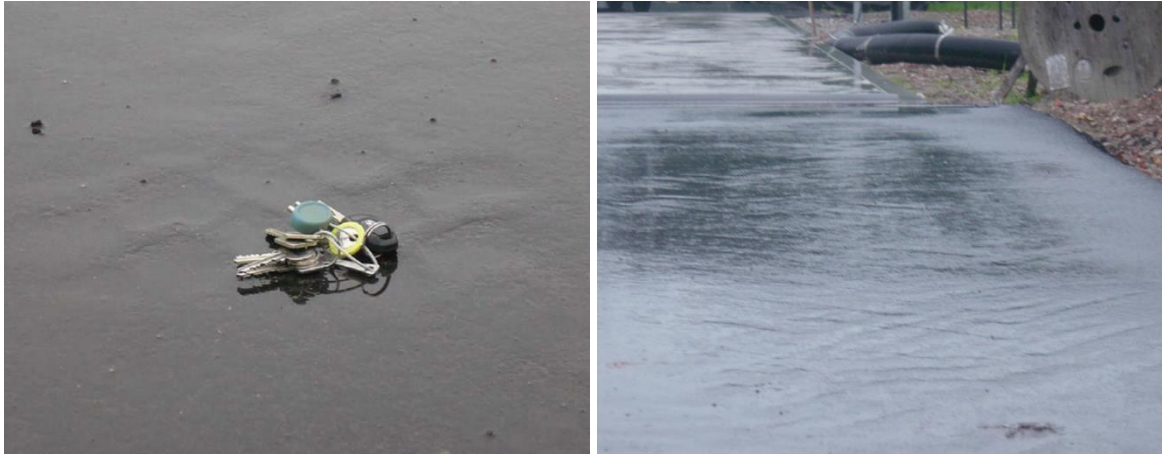
Figure 3. Light marks in the surface layer (Ohe & Behle 2012)
