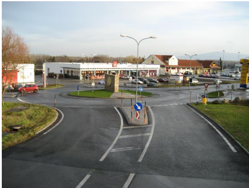
Figure 12. KV Hainburg on the B 9 federal state road/Kruecklstrasse in Hainburg (Province of Lower Austria) (Hrapović 2016b: 280)
