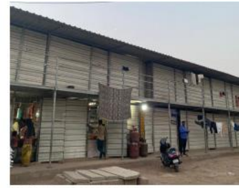
Fig. 37 : View towards first block
