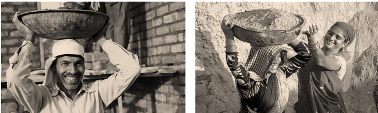
Figure 4. Workers at construction sites
