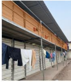
Fig. 34 : View showing double storey units
