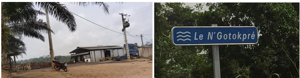
Photo 2: Overview of the oil mill installed on the Baffia road
