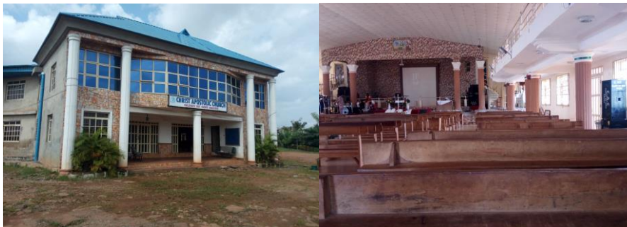
Plate 4: Main entrance and interior space of to the CAC Glory of God church Source: Researcher’s field work, 2018
