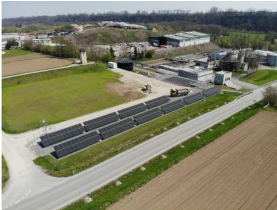
Figure 8: Photovoltaics and combined heat and power plants (Germ. BHKW – Blockheizkraftwerk) cover the energy needs of the Ager-West sewage treatment plant (HIPI, 2022)
