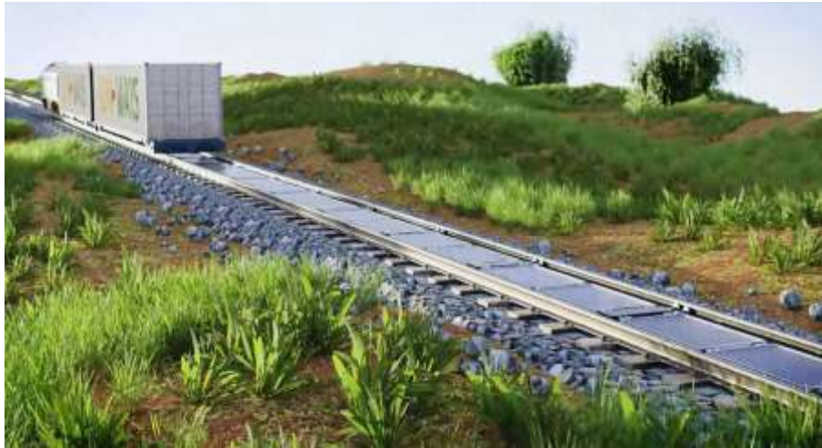
Figure 16: Sunways wants to use a special train to roll out the solar modules between the rails, as a 3D animation by the start-up shows (Koch, 2023)
