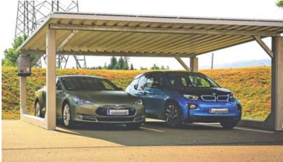
Figure 12: Due to the special prefabricated concrete parts, no foundations are necessary (WKA ÖKOSTROM GMBH, 2023)
