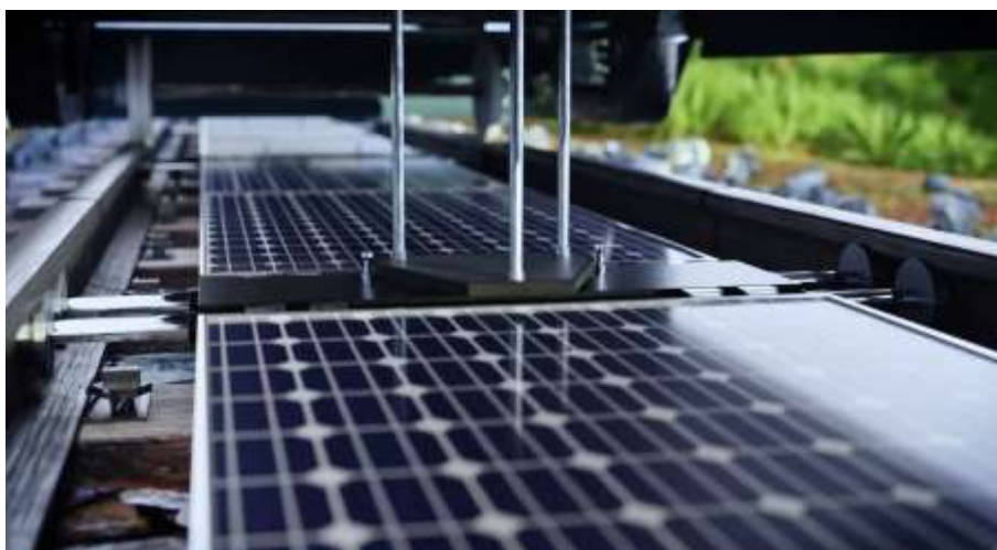
Figure 17: The special pull is to trigger a mechanism that fixes the panels in place (Koch, 2023)
