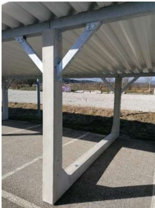
Figure 15: Parking spaces at Star Movie in Regau are covered with a huge photovoltaic system (Hrapović, 2023)
