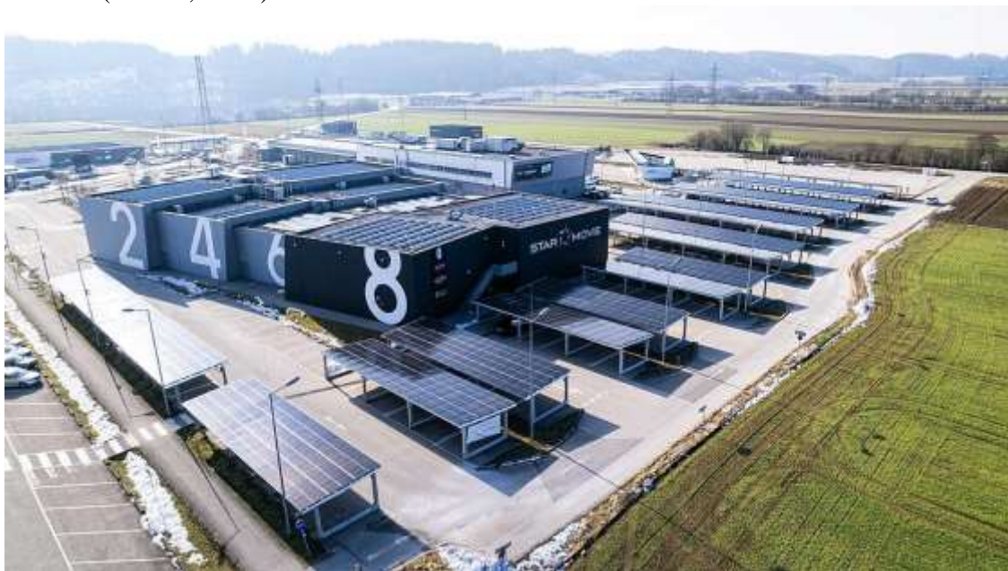
Figure 11: The covered cinema parking spaces in Regau produce electricity for 140 households. Image: Starmovie (free of charge) (Brandner, 2023)
