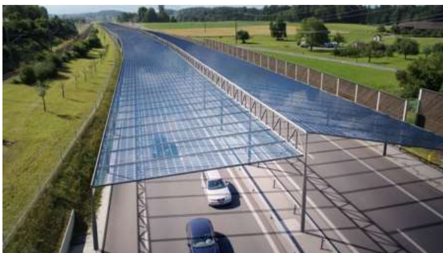
Figure 5: This is what a photovoltaic roof for highways should look like one day (Hrapović, 2022; Nefzger, 2020)
