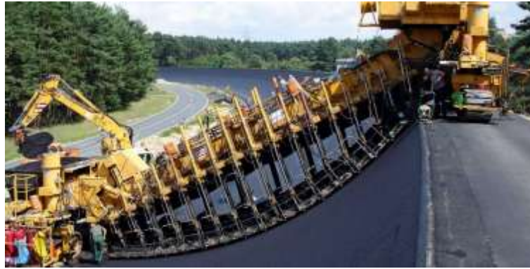
Figure 22. Asphalt paving of the parabolic surfaces by special bridge paver 3
