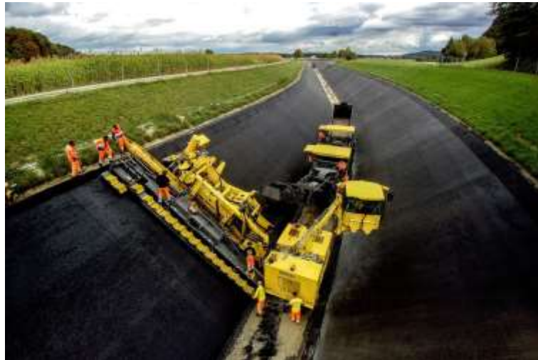
Figure 6. Paving with a bridge paver in a water channel 1
