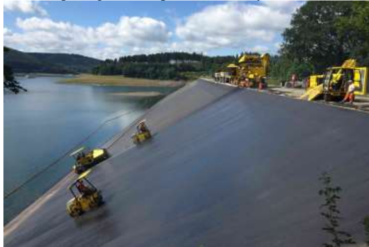
Figure 20. Installation of the asphalt surface course 1
