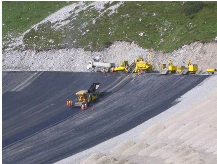
Figure 13. Most of the mix was brought to the site by 4-axle truck (Danklmaier, 2008)
