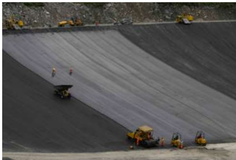
Figure 18. Reservoir Seekar at Zauchensee: Installation of sealing layer 8,700 to (Danklmaier, 2008)
