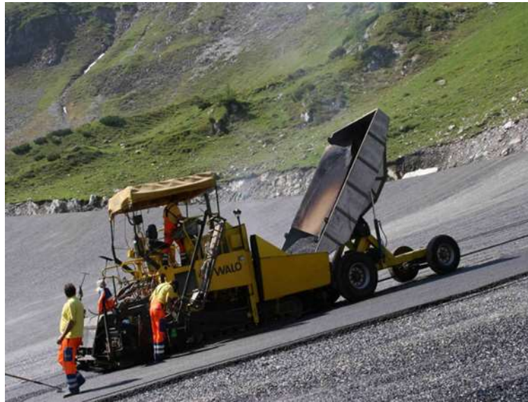
Figure 15. Transport of the mixture with paver charging wagons (Danklmaier, 2008)
