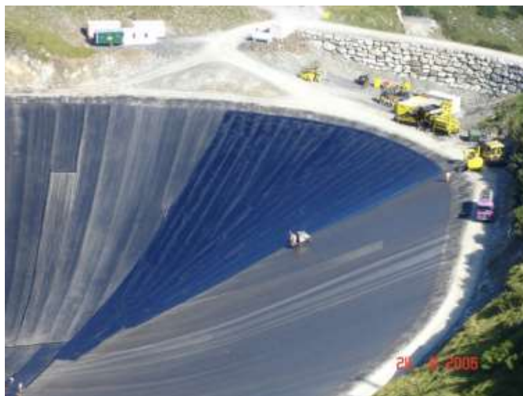
Figure 19. Reservoir Seekar at Zauchensee: Installation of mastic (Danklmaier, 2008)
