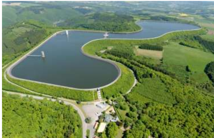
Figure 2. Upper reservoir of the Vianden pumped storage power plant in the Grand Duchy of Luxembourg 2
