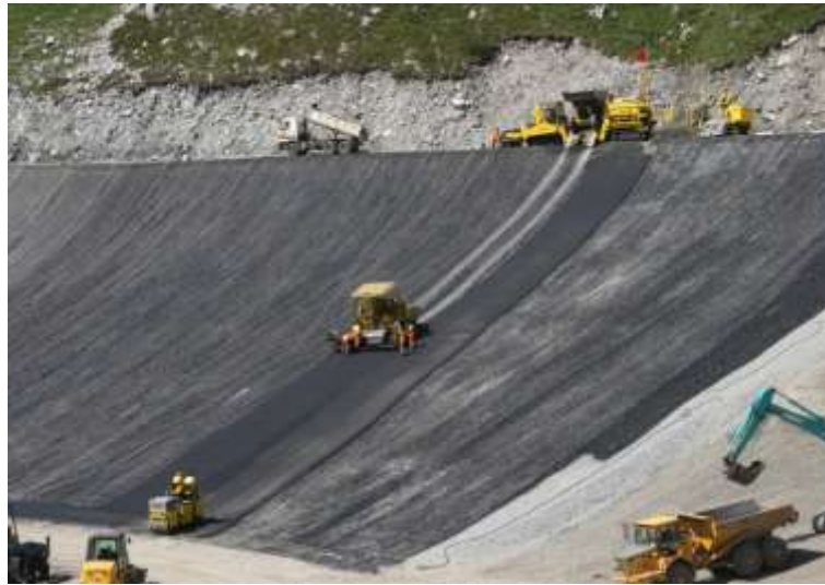
Figure 17. Paving of binder course 9,700 to (Danklmaier, 2008)
